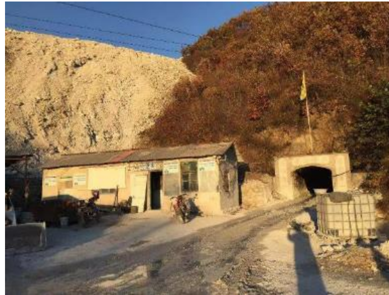
Entrance to Mine
