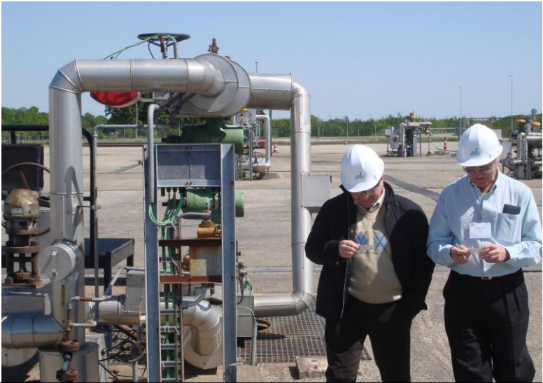
Nedmag's Mg-salts solution mine, Veendam, the Netherlands
