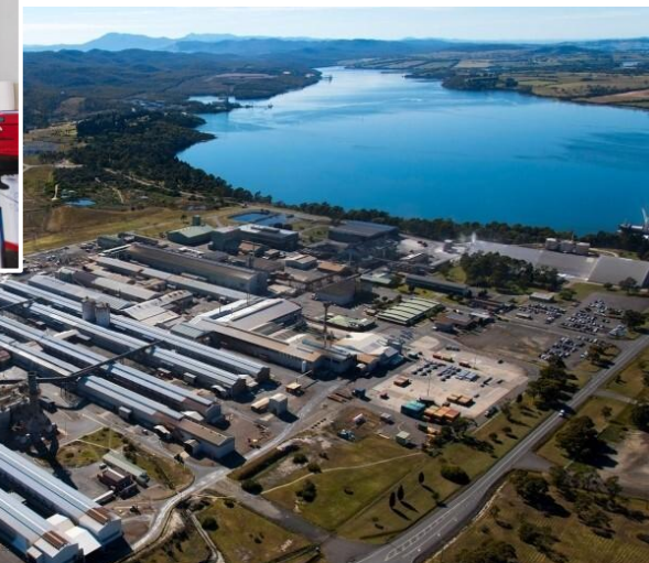
ALCORE pilot plant using Al smelter waste from Rio Tinto Bell Bay, Tasmania
