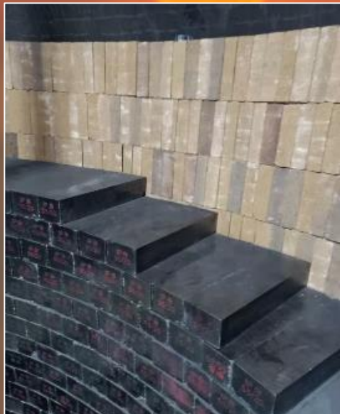
Lining refractory bricks at Benxi Steel Group, Benxi, Liaoning, China
