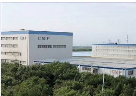
CMP Main Plant
